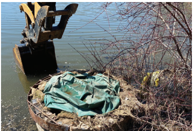
BEFORE: CONTROL STRUCTURE PLUGGED
