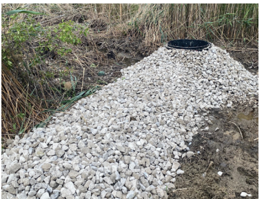
BEFORE: CONTROL STRUCTURE PLUGGED
